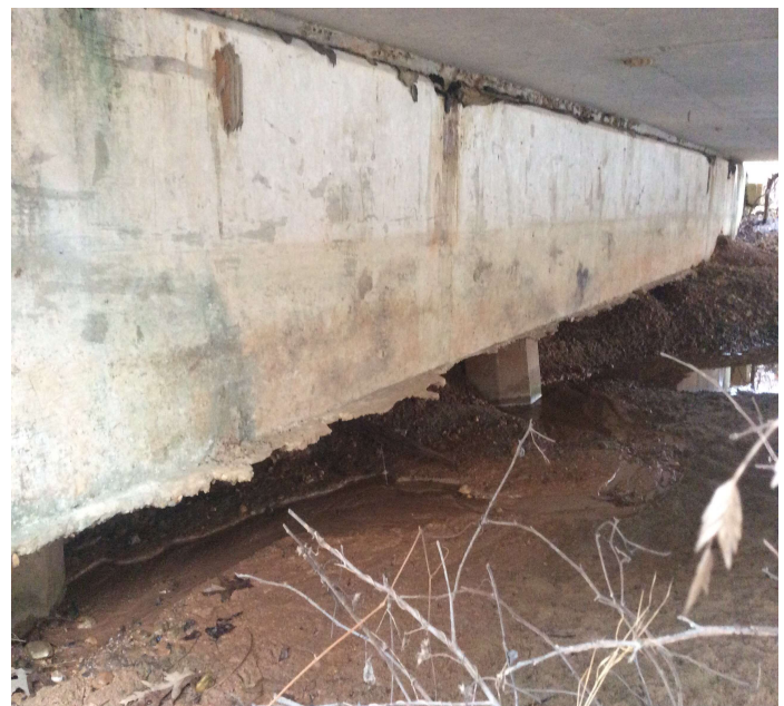
PHOTO 2 Description Abutment 1 cap, scour back under the abutment cap with minor roadway settlement.
