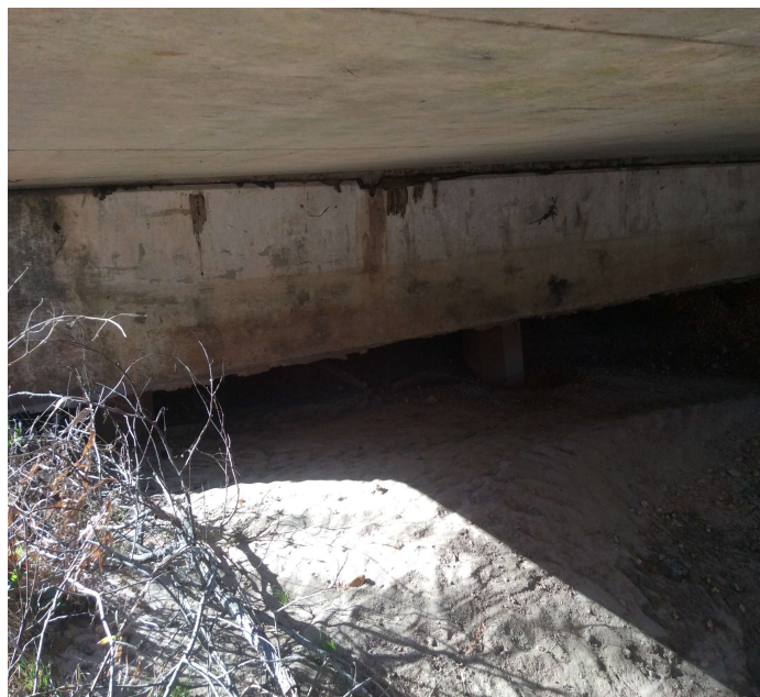
PHOTO 1 Description Minor washing abutment 1
