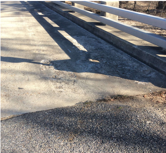
PHOTO 1 Description Spall span 1 right.
